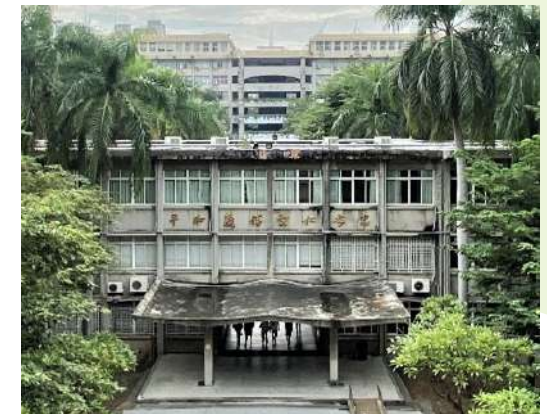
Exterior view of the University Archives - Northern Building, Jiangong Campus
