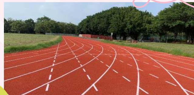
PU track improvement at the First Campus
