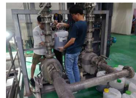
Carbon Neutral and Energy Technology Research Center
