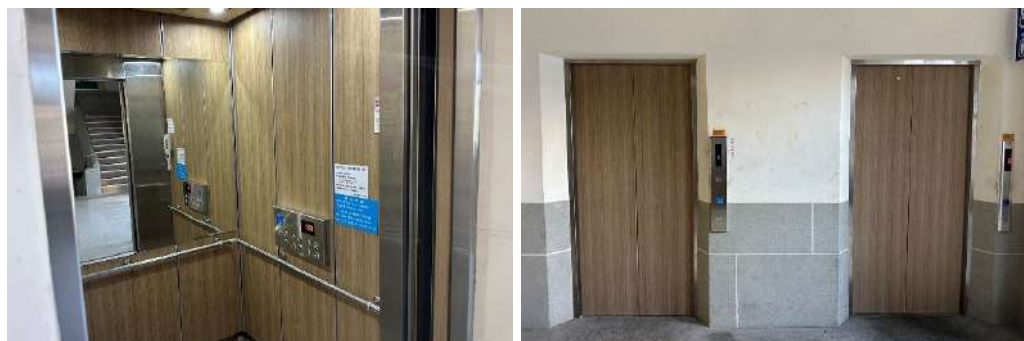
▲ Replacement and Upgrade of the Accessible Elevator in the Student Activity Center on the First Campus
