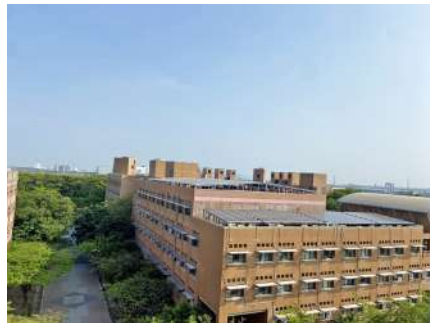
▲ Rooftop Solar Photovoltaic System on the College of Electrical Engineering and Computer Science Building, First Campus
