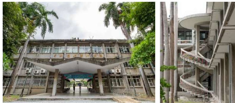
▲ The North Arcade, Connecting Corridor, and W-Shaped Folded-Plate Canopy on the Northern Façade, and the Semi-Circular Spiral Staircase on the Southern Façade – North Building, Jiangong Campus
