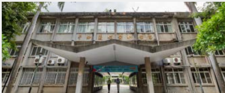
▲ North porch, corridor, and W-shaped folding panel canopy
