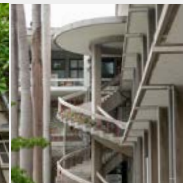
▲ Semi-circular spiral staircase on the south elevation
