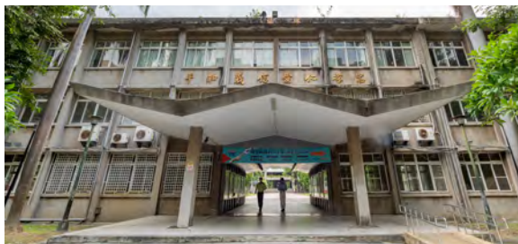
▲ North porch, corridor, and W-shaped folding panel canopy
