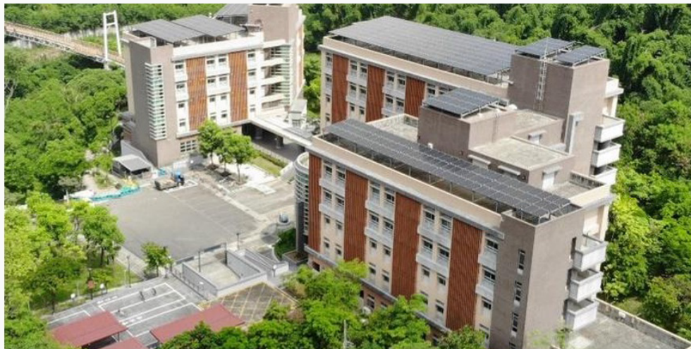
▲ Yanchao Campus Dormitory Solar Power System
