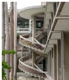
▲ Semi-circular spiral staircase on the south elevation
