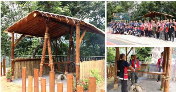
▲ The 'volunteer construction' team created the 'Sustainable Na-House' for Minsheng Elementary School
