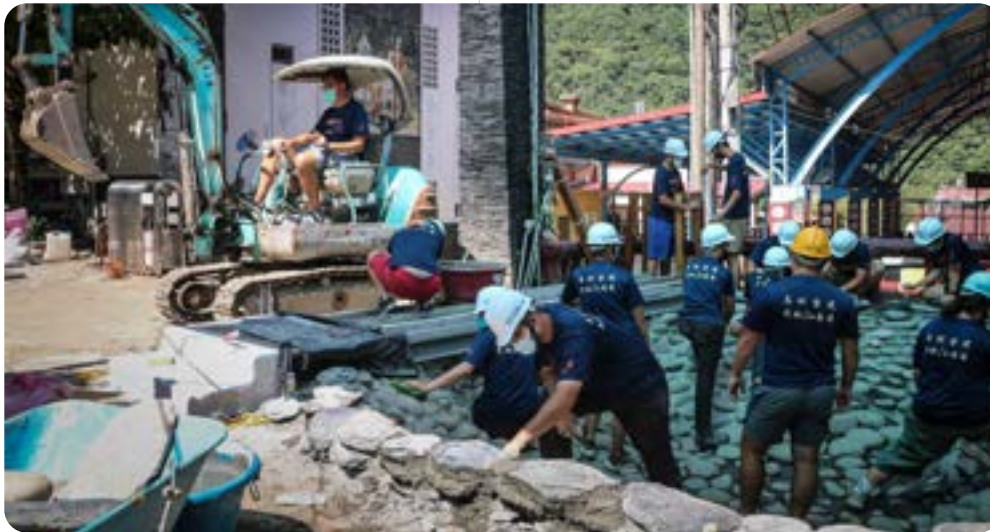
▲ Ecological pool construction process
